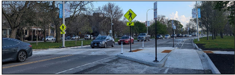
A bike lane and speed bump recently constructed in Humboldt Park.
