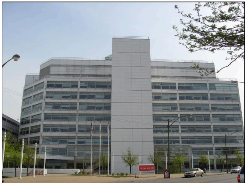
The Cook County Juvenile Temporary Detention Center located on the Near West Side of Chicago.
